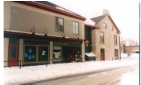
Colbourn Street Facade
